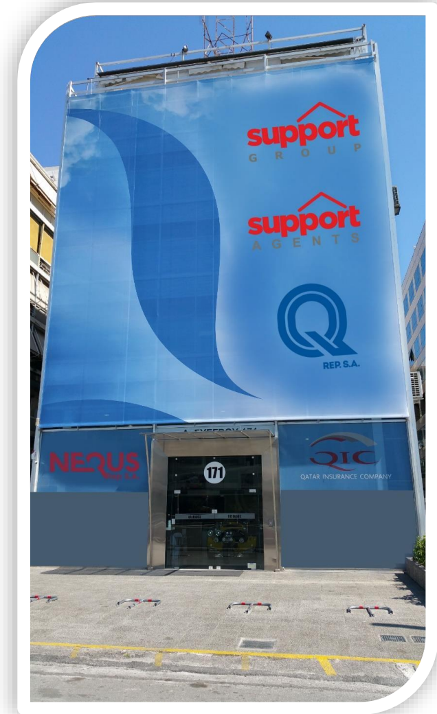
The Building at 171 Syngrou Ave. in Nea Smyrni, which houses the Nequs Rep S.A. company.
